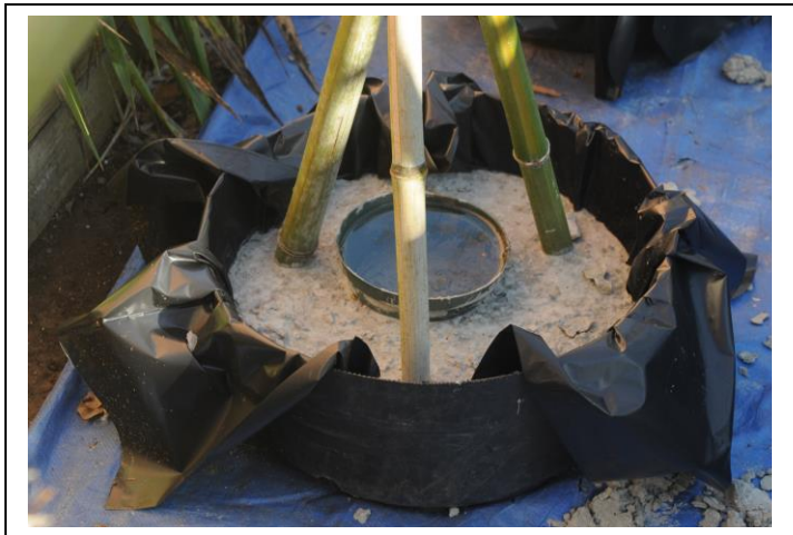
Tripod with hole. The garbage bags held the Quikrete while drying and covered the “whiteness” when Spanish moss was added to top.
